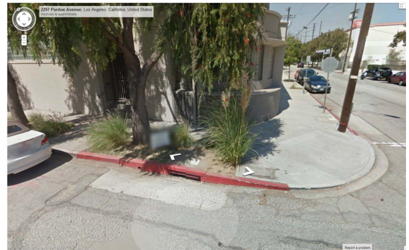
Nearest Catch basin on Purdue St. One and half block away
