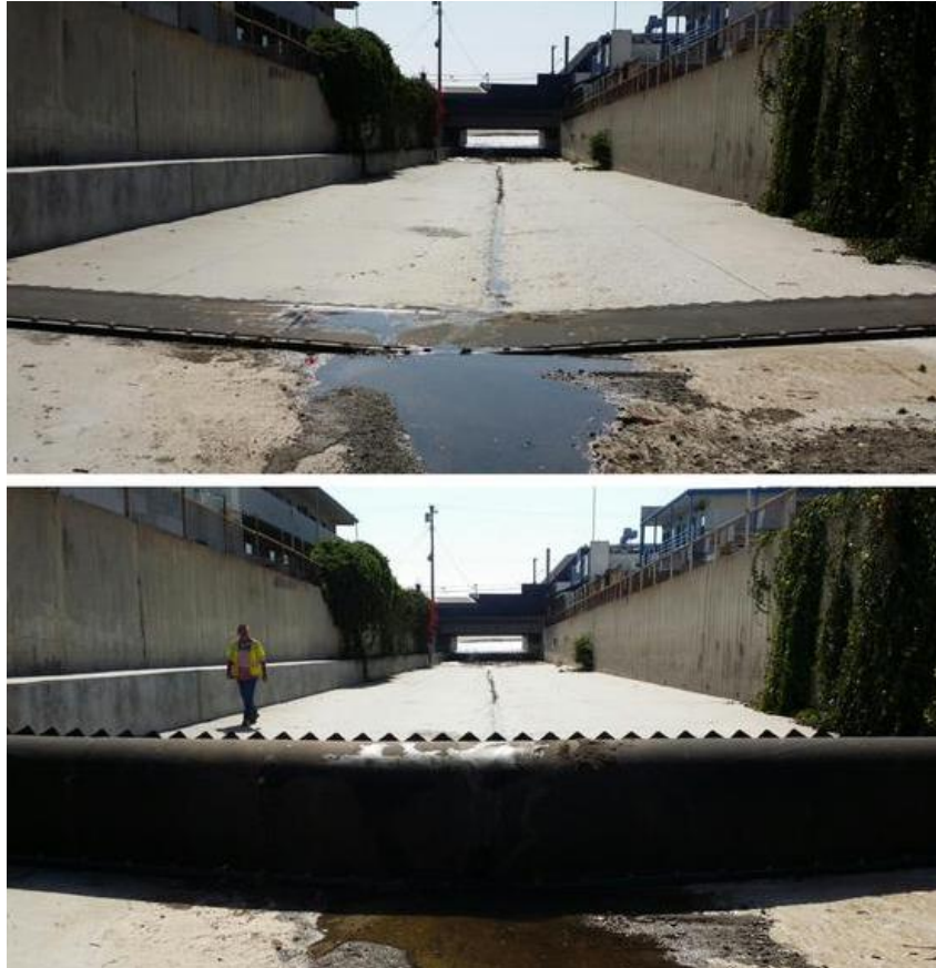
Figure 5. Rubber Dam Diversion in Santa Monica Canyon downstream from Riviera (photo credit: Josh Svensson)
